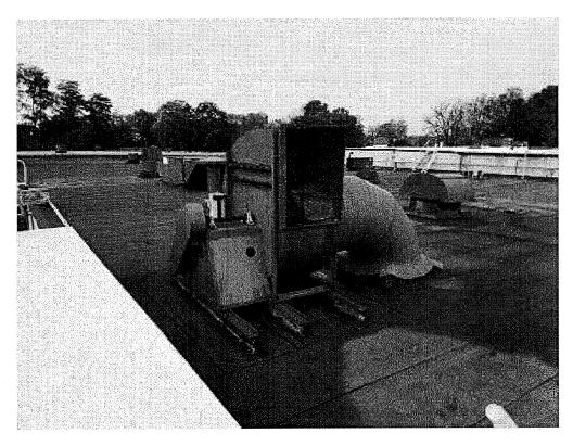
Image 3(Roof Exhaust): Roof exhaust from etch tank line
