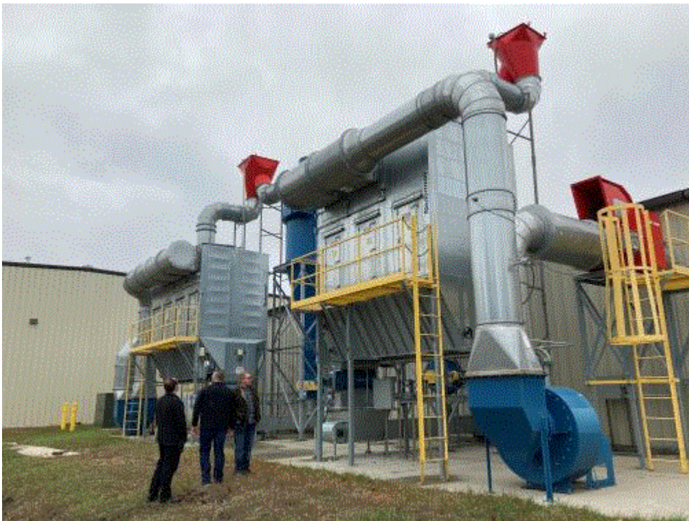
Image 3(EUEXTRUSION2) : Cyclone and Bagless Baghouse of the EUEXTRUSION2 process.
