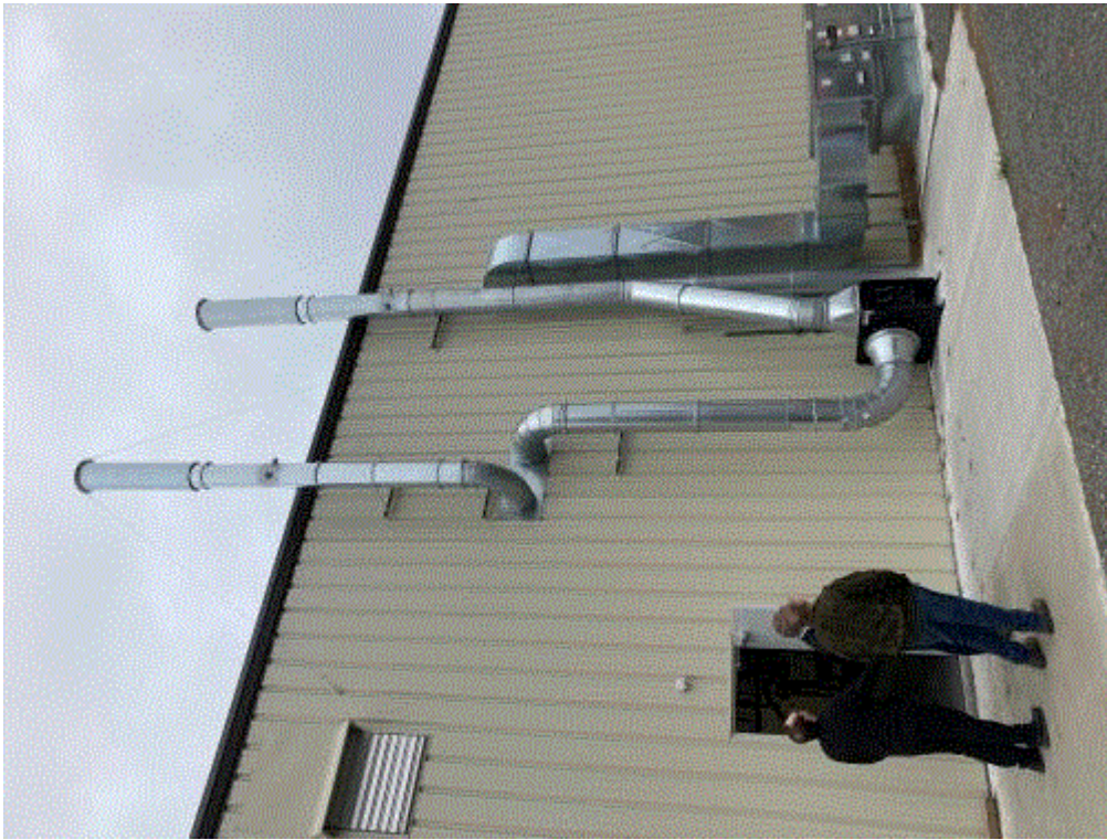
Image 6(EUFLORALFOAM) : Exterior view of stacks. Left is chemical storage locker, and right is the oven hood vents, and then you can see the heating/cooling duct work.
