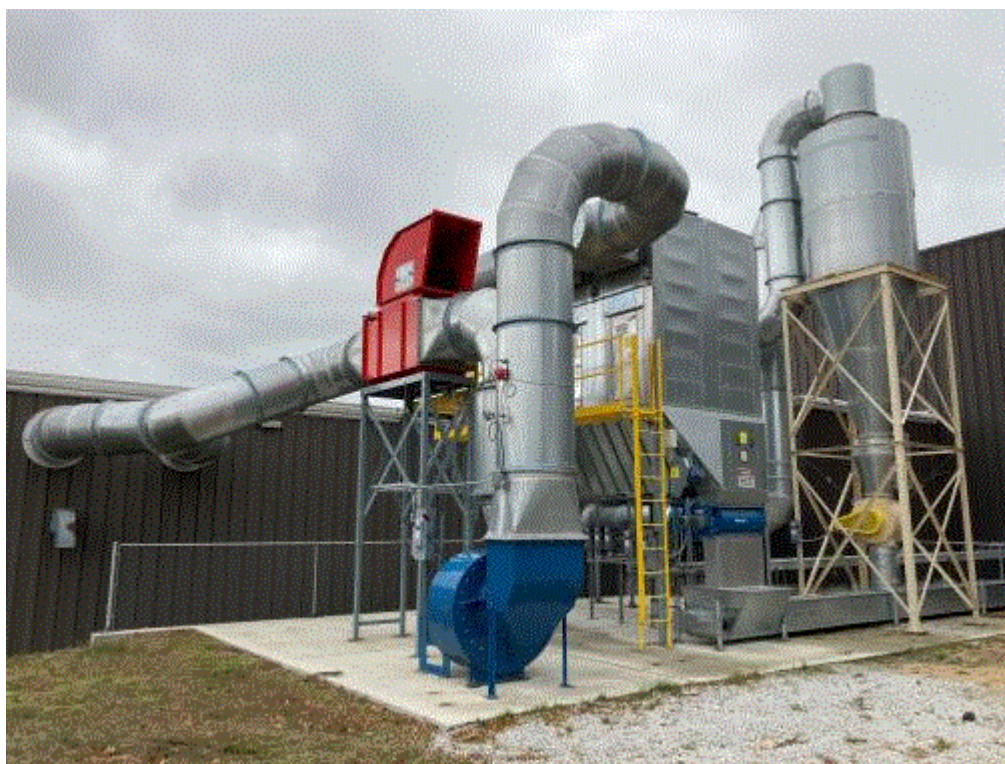
Image 1(EU EXTRUSION1) : Cyclone and Bagless Baghouse for EU EXTRUSION1 process.
