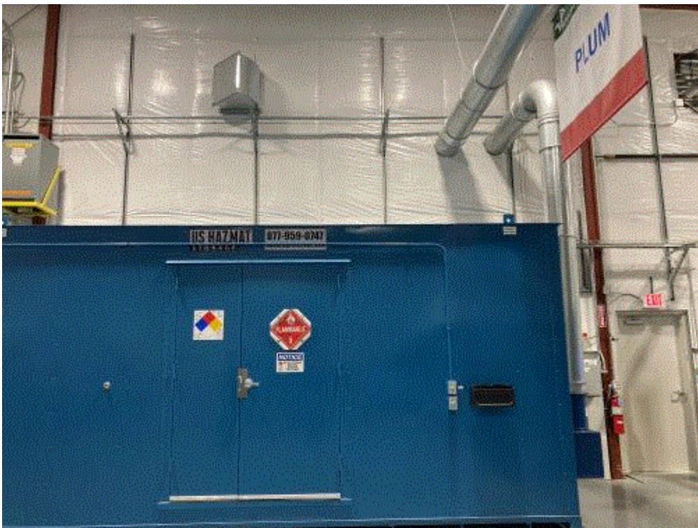
Image 5(EUFLORALFOAM) : Chemical Storage Locker and view of stacks exiting the building. Center - Heating and cooling vent. Round Stack on Left - from oven hood vents. Round stack on right - Chemical storage locker.
