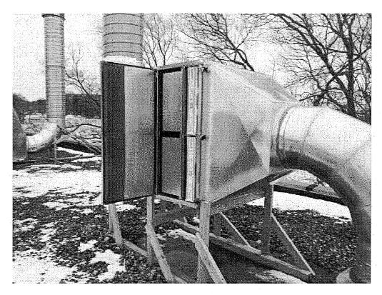
Image 1(Open Stack) : GAC and PM filters
