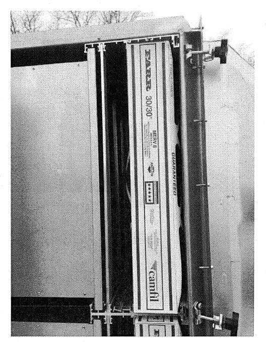
Image 3(PM filter) : Camfil brand particulate filter (right) and GAC tray (left).
