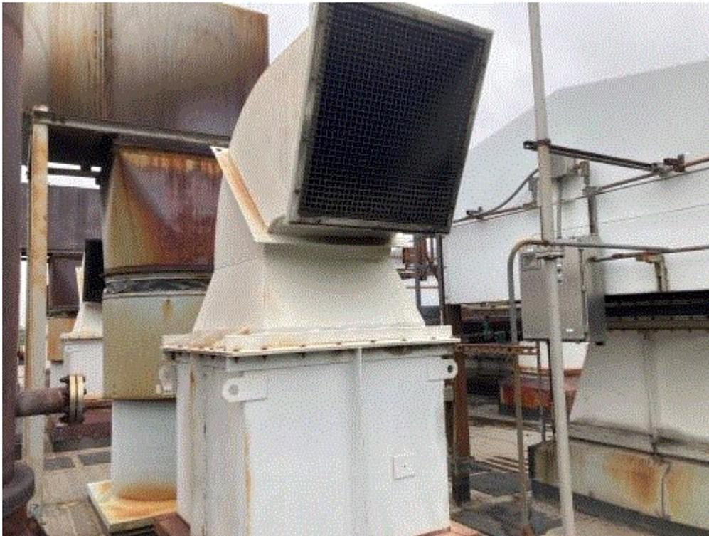
**Image 1(Cooling Stack)** : Turbine cooling stack on roof of turbine building
