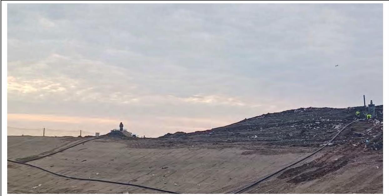
**Photo #4 – View looking from the northwest showing 6-inch vacuum lines installed to wells AHWW0539 and AHWW0540**
