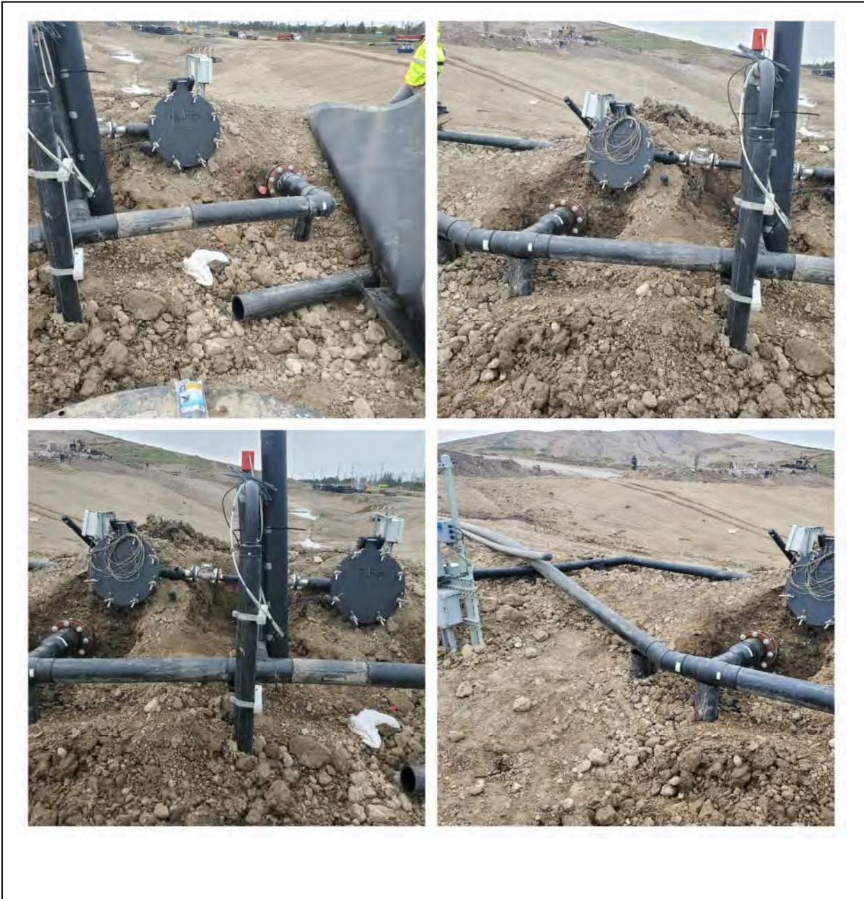
**Photo #1 – 6-inch pipe and vacuum line connections made to 3 leachate clean-out risers prior to installation of liner cover installation.**
