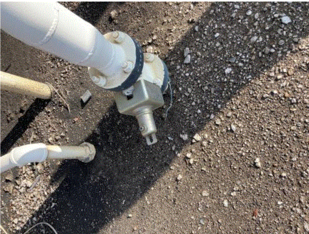
Image 2(Gas Lock) : The Lock on the gas line to the Lime Dryer.
