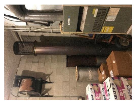
Image 2(Stack) : The dismantled stack where unit once was. Ceiling can be seen to have been closed since removal of stack.
