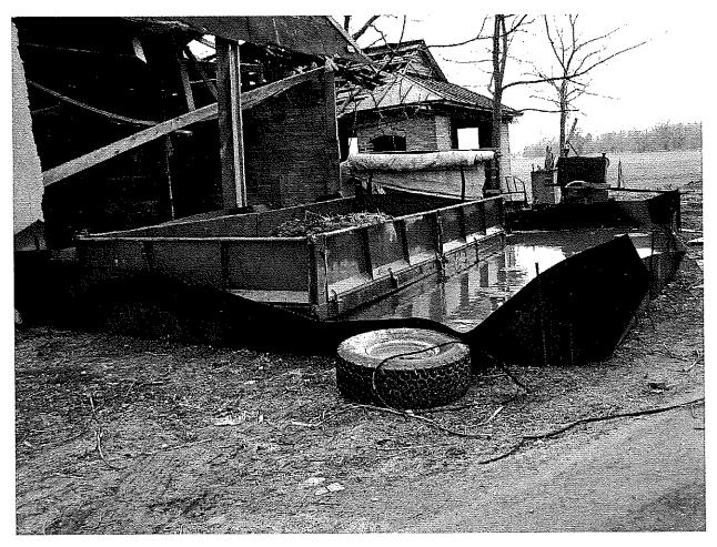
Figure 3 Red dumpster with what appeared to be contaminated soil. Photo taken over concerns about the integrity of the secondary containment that is filled with water.
