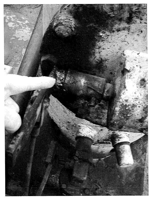
Figure 2 Closeup of EUNIXON4SEP separator tank for the Nixon 4-23 sour well. The hole in the piping is indicated at the end of the finger included for scale. H2S reading 82 ppm.
