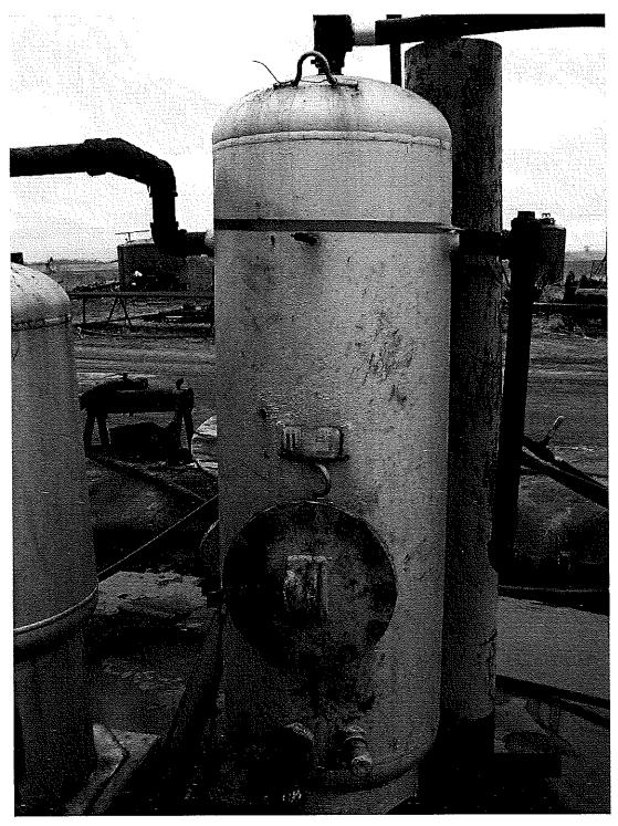
Figure 1 EUNIXON4SEP separator tank for the Nixon 4-23 sour well. Piping near bottom-center-left had a hole and was leaking H2S at 82 ppm.
