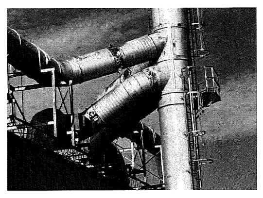
Image 2(central stack) : view of stack and wyse joints for central stack. Note the metallic coating of rubber banding at joins is coming off.
