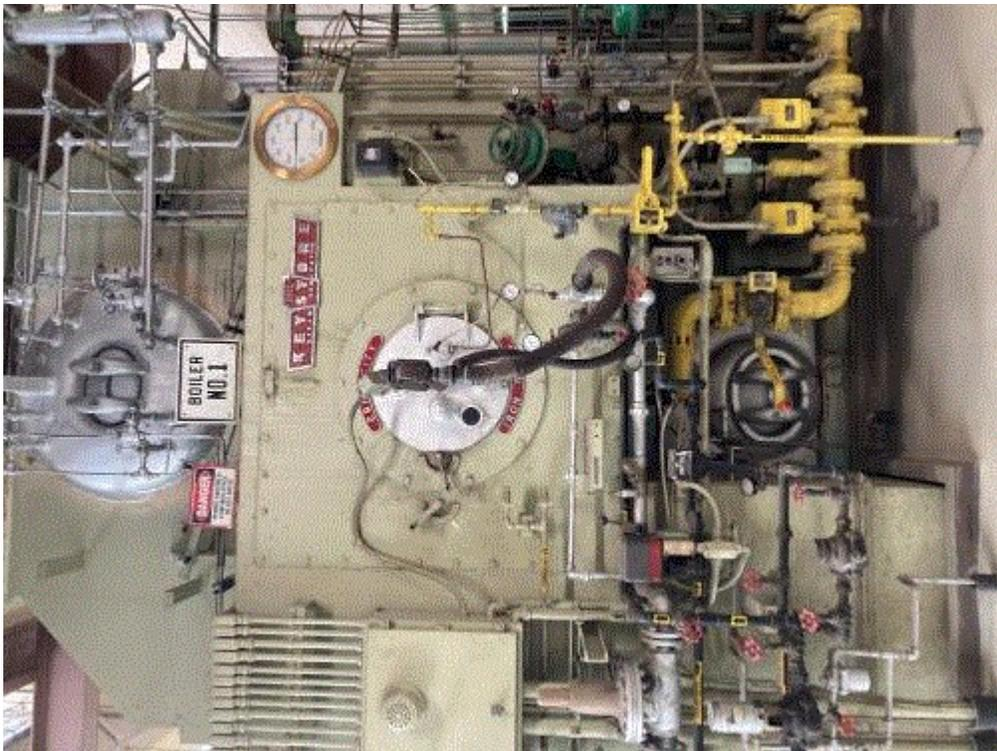
**Image 2(Boiler 2)** : Natural gas fired Boiler 2.
