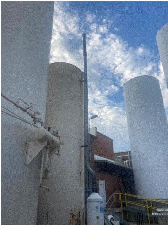
**Image 2(Sludge Tank) :** Photo of the corrected exhaust stack for the sludge tank.
