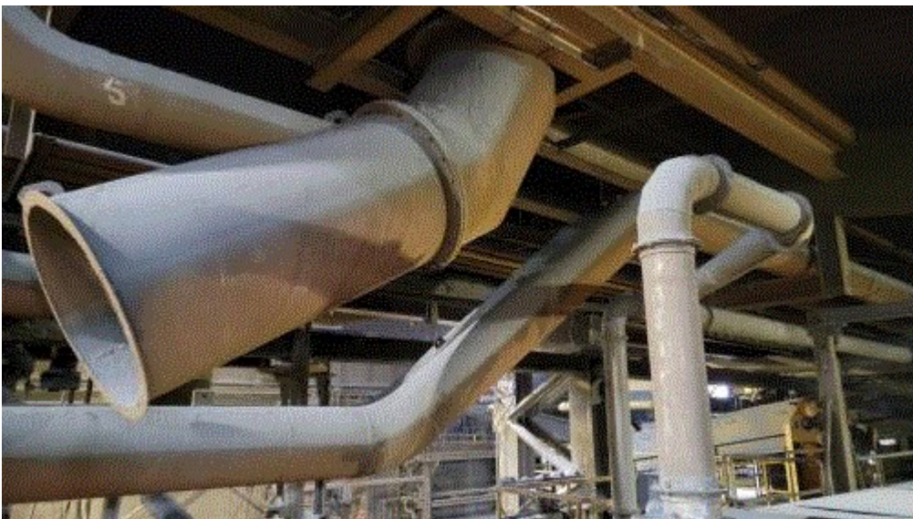
Image 2(EAF Baghouse) : Location on proposed tie-in to the EAF baghouse from the VTD process that is currently ducted into the LMF baghouse.
