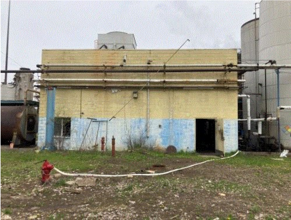
Image 4(004) : Exhaust vent for EUPilotOxidation is pipe at 45 degree angle above roofline, as seen on 5/5/2022.
