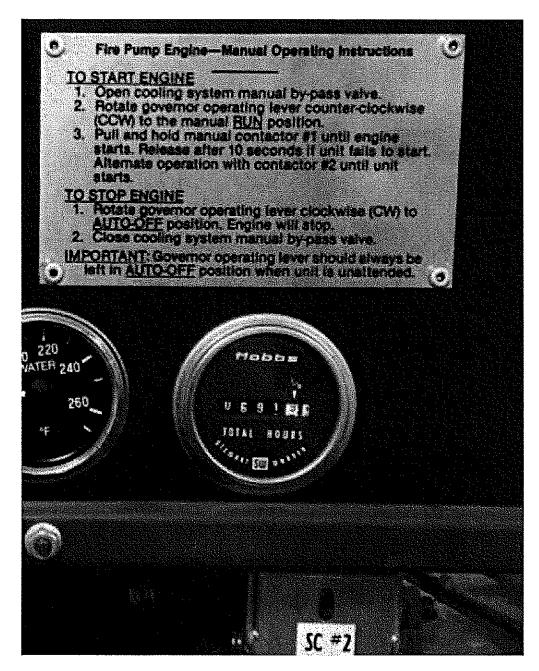
Image 9(9): West Clarke Detroit Diesel Pump 2 - Hour Meter from May 18, 2018. Photo supplied by Duke Couch
