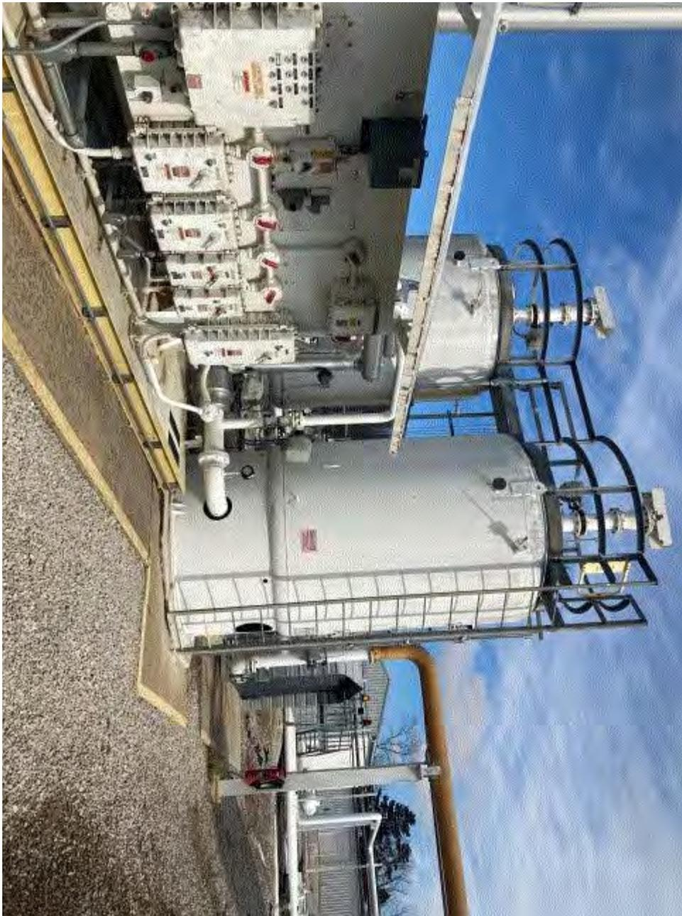
**Image 2(VRU carbon beds)** : Vertical structures house the carbon adsorption beds for VRU
