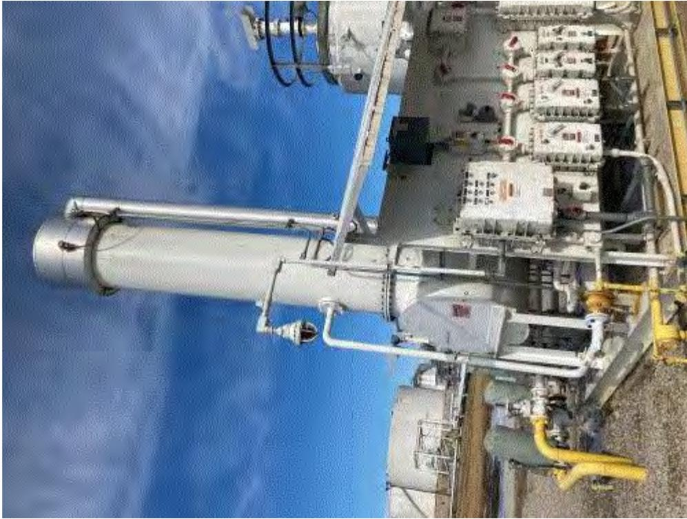
**Image 1(VRU stack)** : Stack for VOC emissions from VRU carbon bed system.
