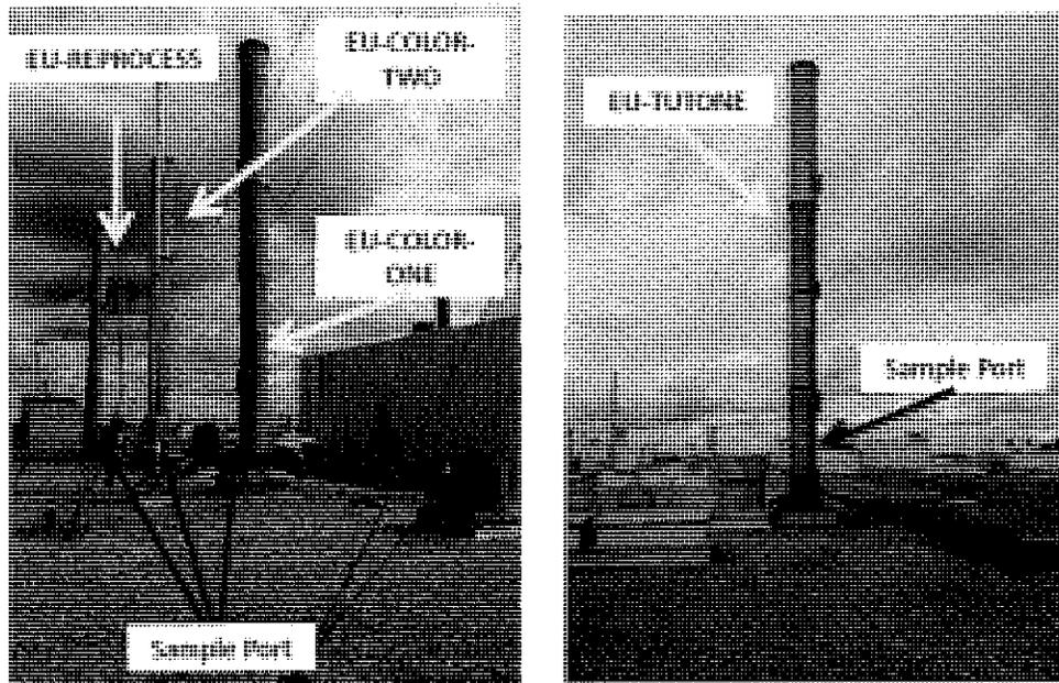
Thermal Oxidizers (TO) Outlet Locations
