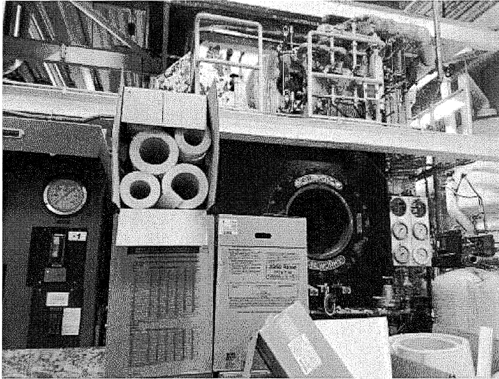
Image 8(Existing Boiler #1) : Existing Boiler #1 (abandon)
