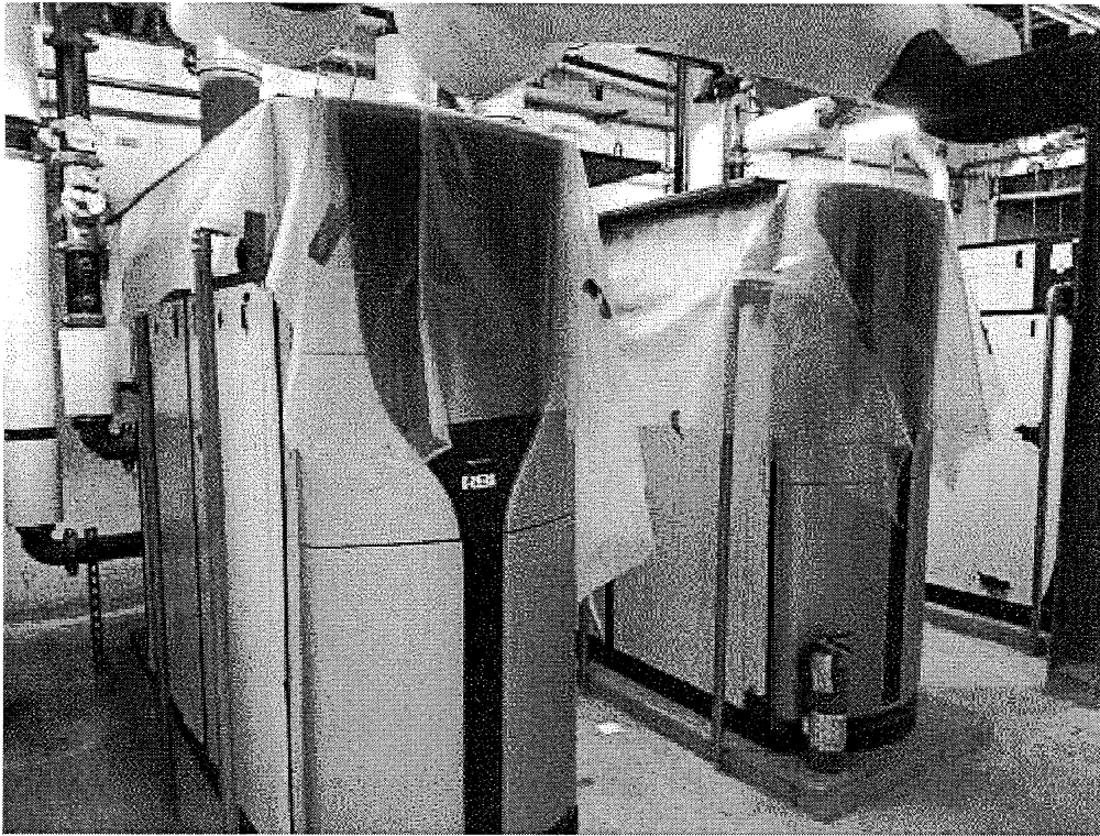
Image 2(Boilers for heating) : Natural gas fired boilers for heating
