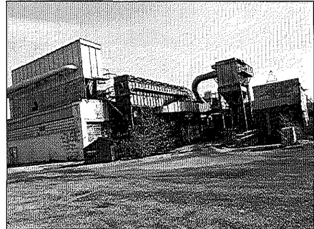
Baghouses serving machining operations (50,000 cfm) Auxiliary collection device to right in photo.
