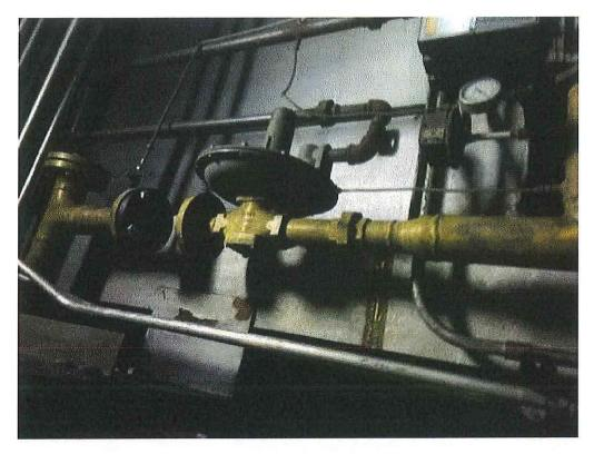
Image 5(EUBOILER3): Disconnected gas line for EUBOILER3.
