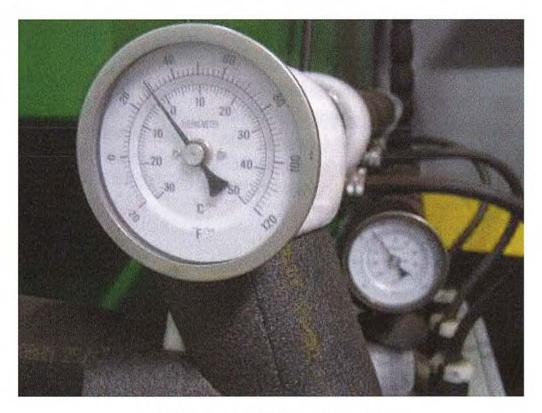
Image 4(004): Chiller inlet temperature gauge.
