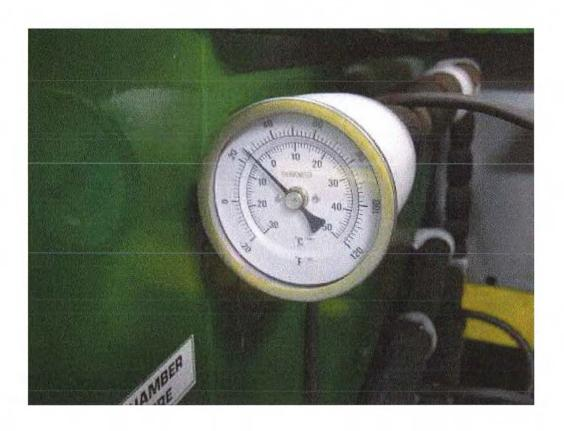
Image 5(005): Chiller outlet for upper level coils.
