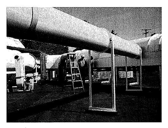
Image 4(Photo 4): Looking N, at 54 inch diam. ductwork (background), to be replaced with twin 24 inch ducts.
