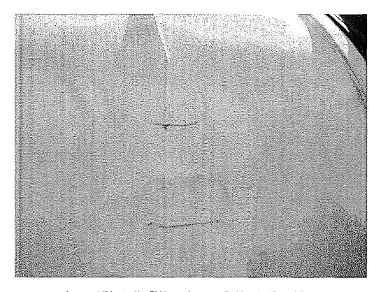
Image 6(Photo 6): PVC patches, applied by plastic welding.
