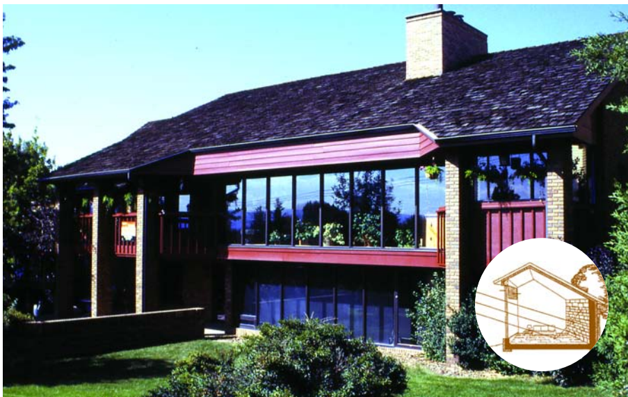
A passive solar home relies on south-facing windows to emit the low-angled winter sun.
