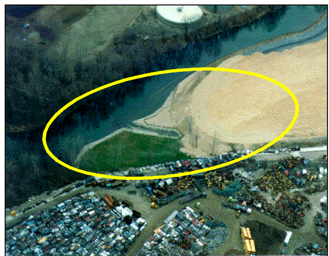
-- Area of Excavation
