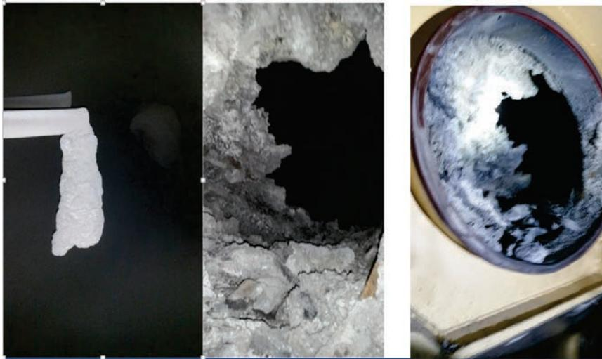
Caustic soda build up on nozzles and the inside of the SDA tower.
