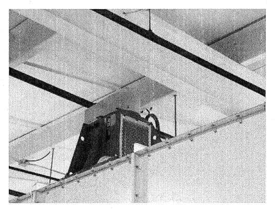
Image 3(Exhaust fan) : Exhaust fan from powder paint booth
