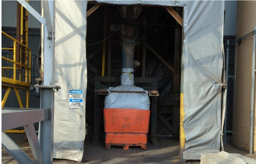
Figure 1. Current Shredder 1 Baghouse Dust Storage Area
