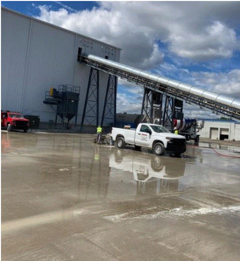
Image 8(Picture 8) : Wet Plant yard
