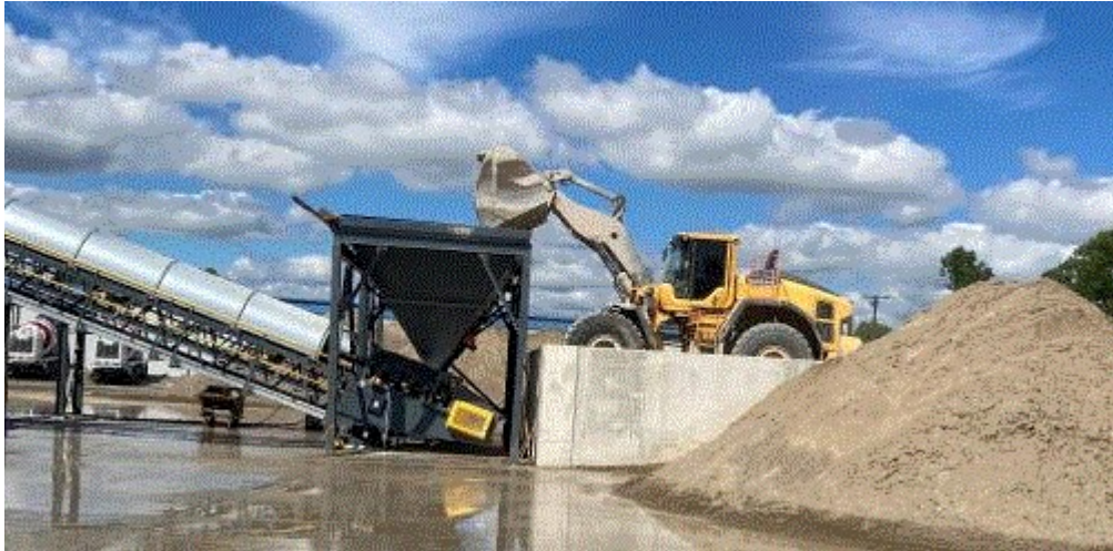
Image 3(Picture 3) : Aggregate transferred to elevated bins through transfer belt and conveyor
