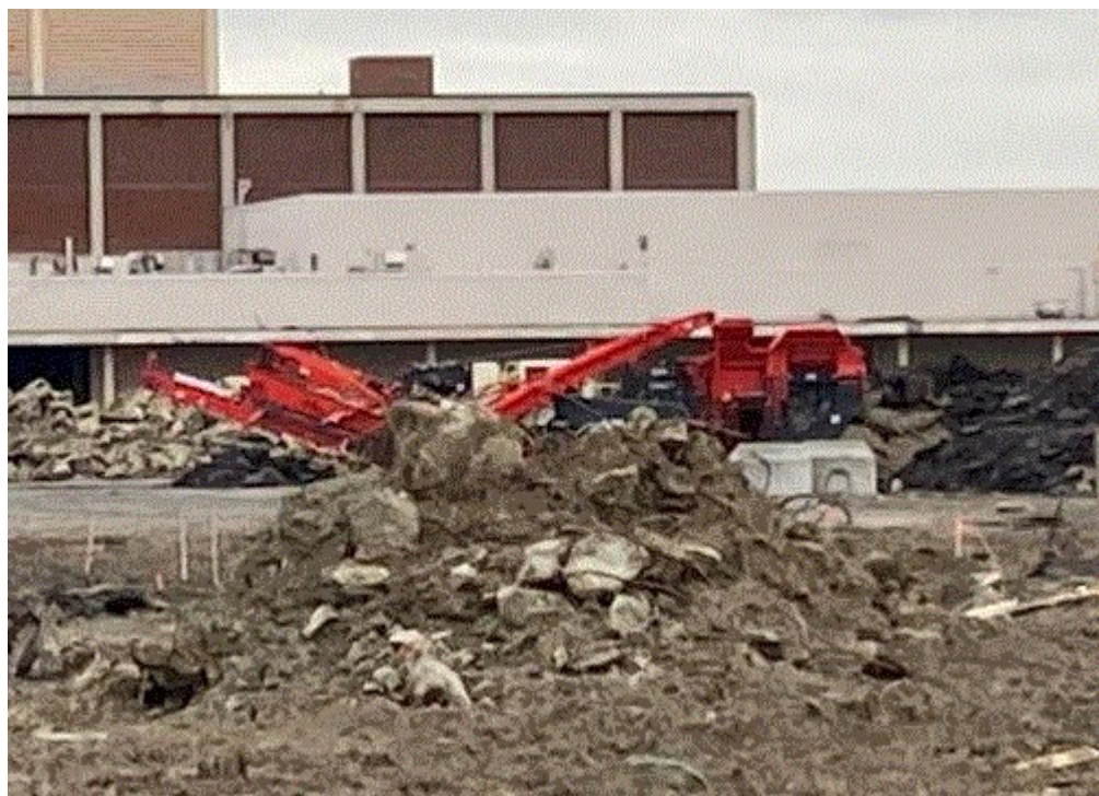
Image 2(IMG 0287 cropped) : Photo of nonmetallic mineral crusher taken by the AQD on 12/15/2021 during an unannounced site observation. The large pieces of asphalt and concrete adjacent to the crusher appear to indicate that this material has not been processed.
