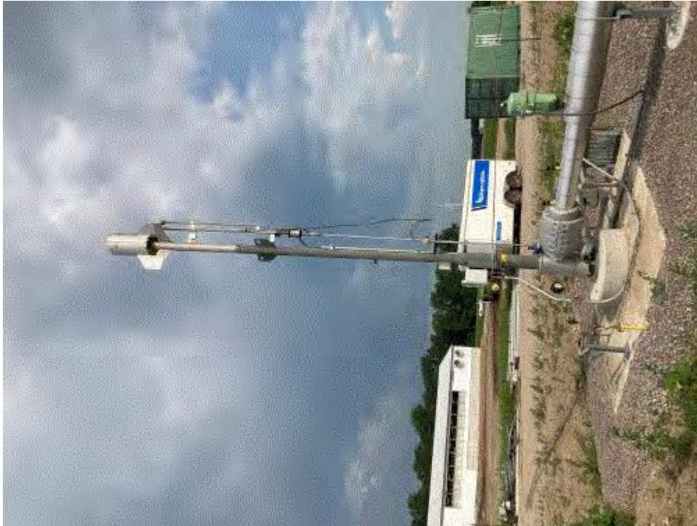
Image 3(Flare) : John Zink biogas flare.
