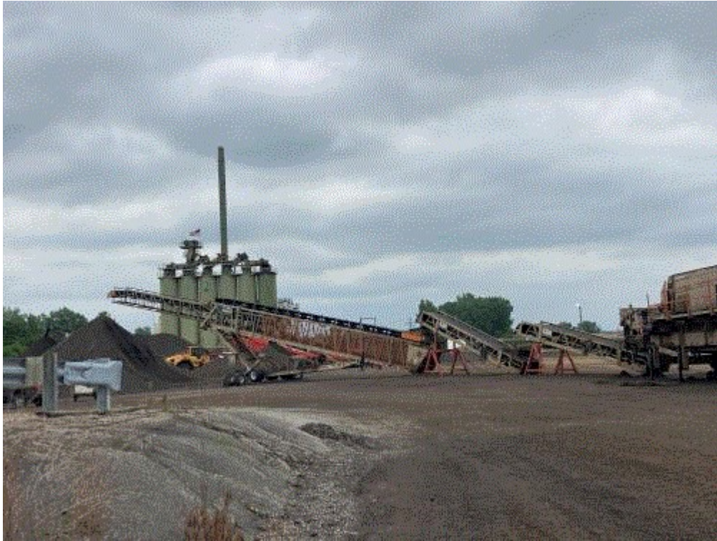
Image 3(KPI JCI) : KPI JCI nonmetallic mineral crushing plant. Asphalt plant in background.
