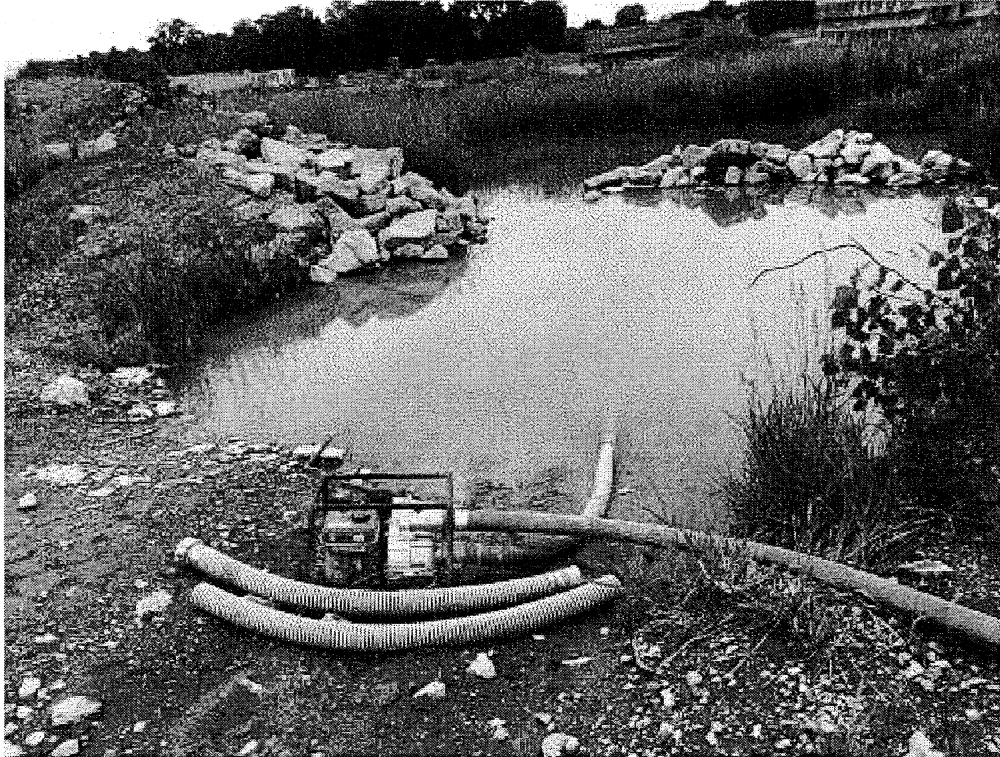
Image 3(water pump) : small water pump and pond at the job site
