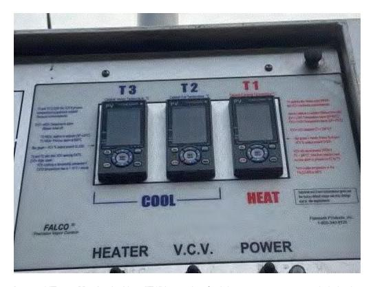
Image 3(Temp Monitor): Note "T1" is monitor for inlet temperature to catalytic bed.
