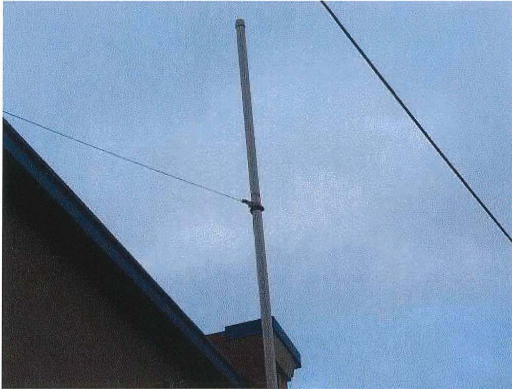
Image 1(20151215 094340 Van) : View of remaining portion of broken exhaust stack. Remaining portion of stack does not meet permit height requirements.
