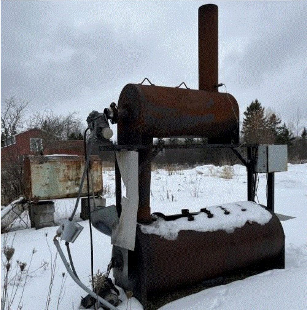
Image 1(Incinerator) : Incinerator shown to be dismantled.
