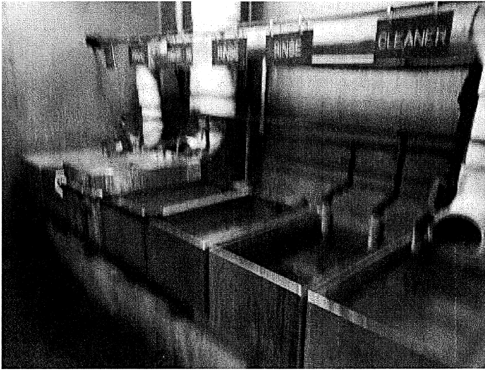
Image 5(Washing/Degreasing) : Washing/Degreasing line.
