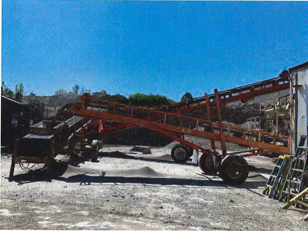
Image 3(Transfer Point) : Conveyor transfer point.
