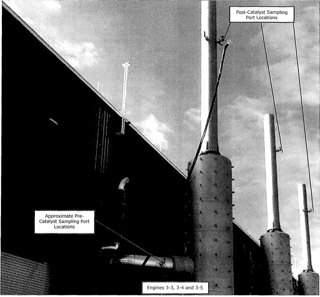
Figure 4-1. Pre- and Post-Catalyst Sampling Port Locations
