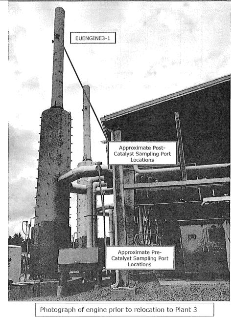
Figure 4-1. Pre- and Post-Catalyst Sampling Port Locations
