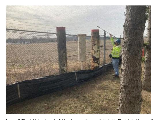
Image 7(Plant 1 blowdown): 3 blowdown vents associated with Plant 1 that had methane emissions.
