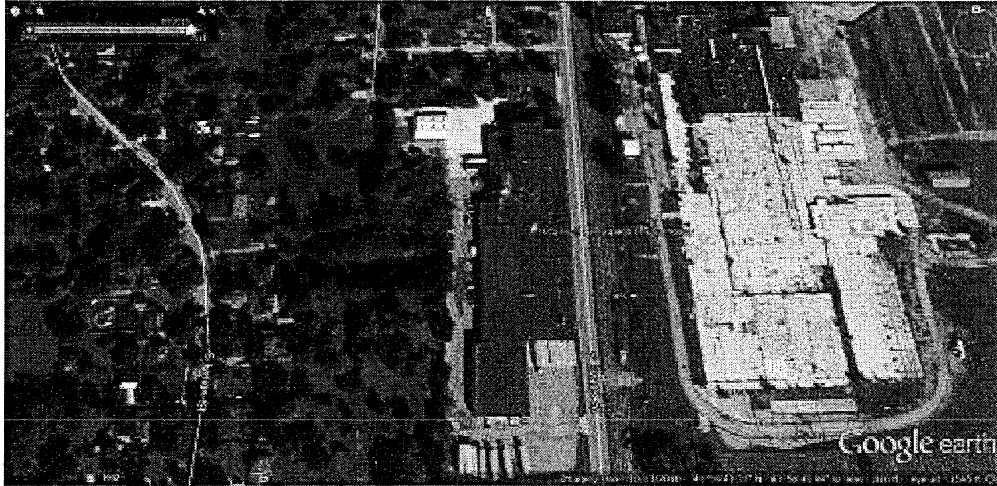
Image 1(aerial photo) : aerial photo
