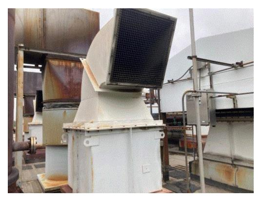
Image 1(Cooling Stack) : Turbine cooling stack on roof of turbine building
