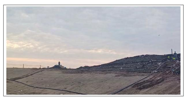
Photo #4 – View looking from the northwest showing 6-inch vacuum lines installed to wells AHWW0539 and AHWW0540
