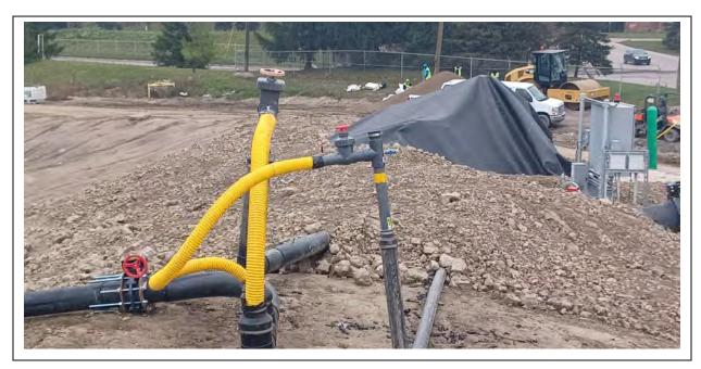
Photo #2 – Liner installed over the leachate cleanout risers to address the penetrations. 3-inch vacuum line installed under liner to maintain negative pressure.
