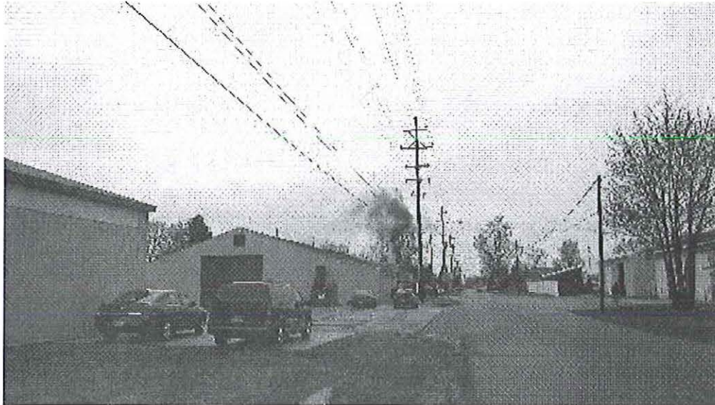
Image 1(View from McBride) : Overview of opacity from McBride Street which is East of the facility. The furthest stack or Unit #2 was the stack exhibiting opacity. glm
