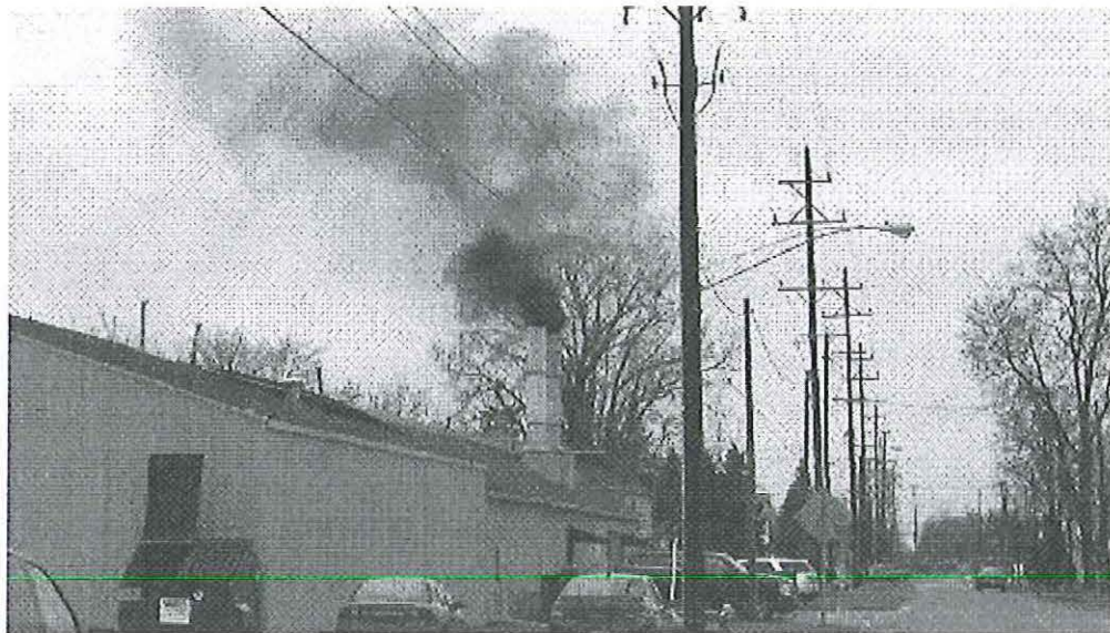
Image 3(Looking West 2) : Additional picture of opacity on Unit #2, looking West towards the facility. Time taken 10:06. glm
