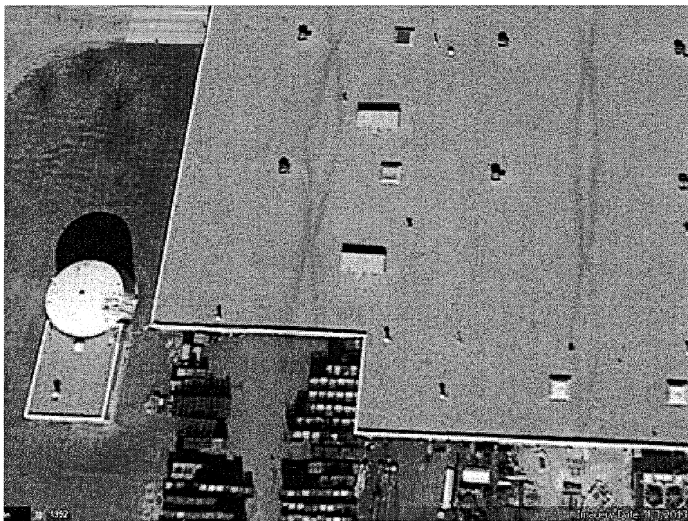
Image 1(4-3-2013 Roof Photo) : Attachment (1) Roof aerial photo taken from Google Earth dated 4-3-2013
