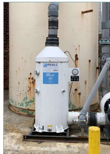
Graphic 6 – Carbon Canister on Sludge Tank Stack
