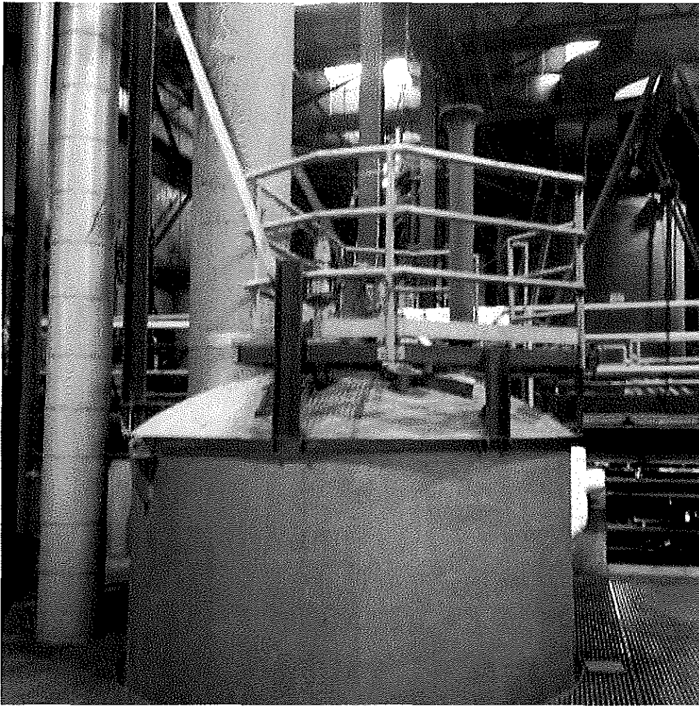
Image 3(Sludge incinerator) : Old sludge incinerator
