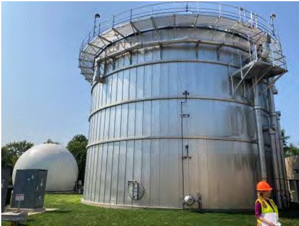
Image 2(Anaerobic Digester) : Photo credit: Erica Shuff. Anaerobic digester.
