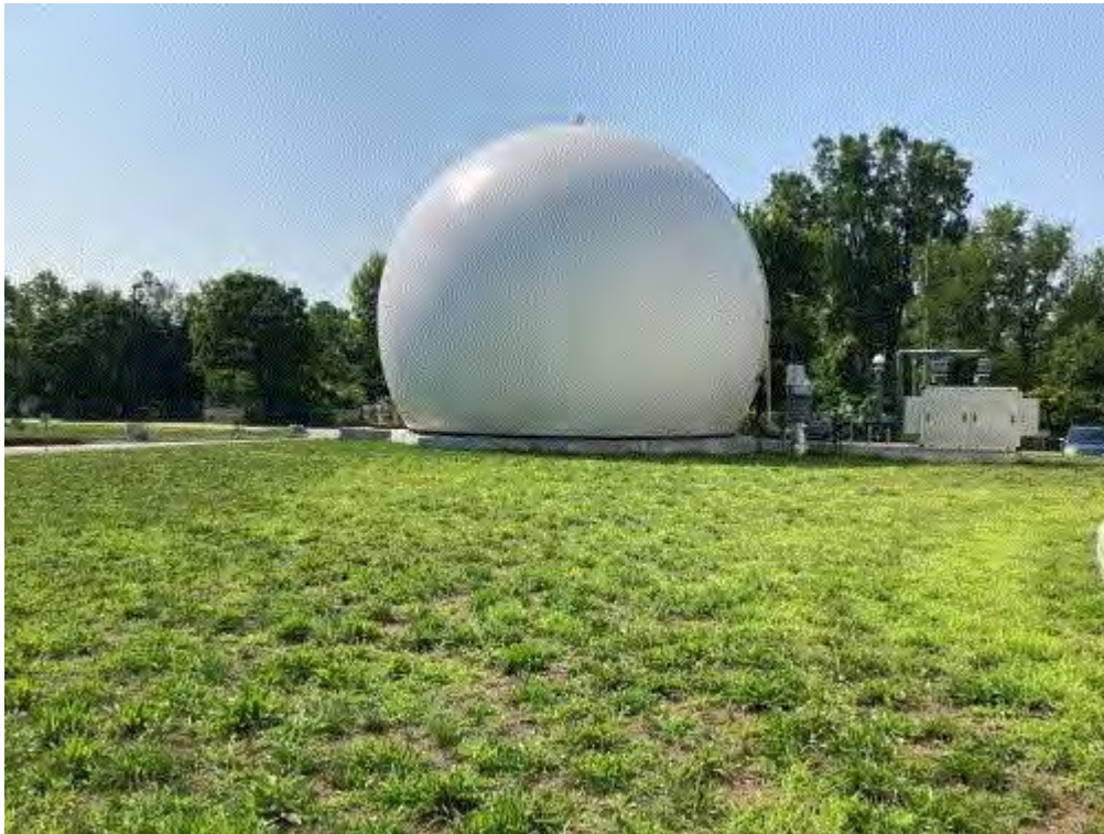
Image 1(Gas Storage) : Photo credit: Erica Shuff. Digester gas storage "bubble"
