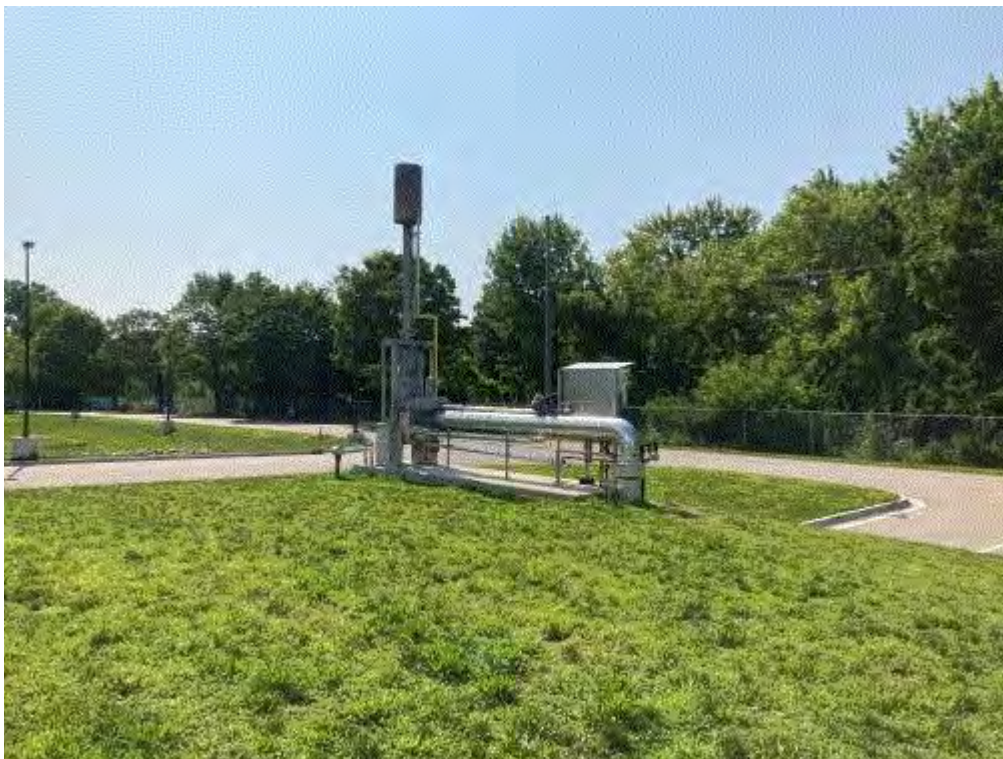
Image 3(Flare) : Photo Credit: Erica Shuff. Open flare for burning sour gas
