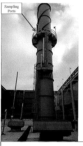
Figure 2-4. SV-MAIN1 Exhaust Stack
