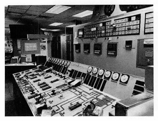
Image 3(056) : Locked Out/Tagged control room at Eckert Station
