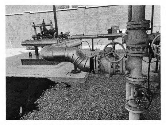
Image 2(048) : Main gas line into REO Town Plant and meter (in blue)
