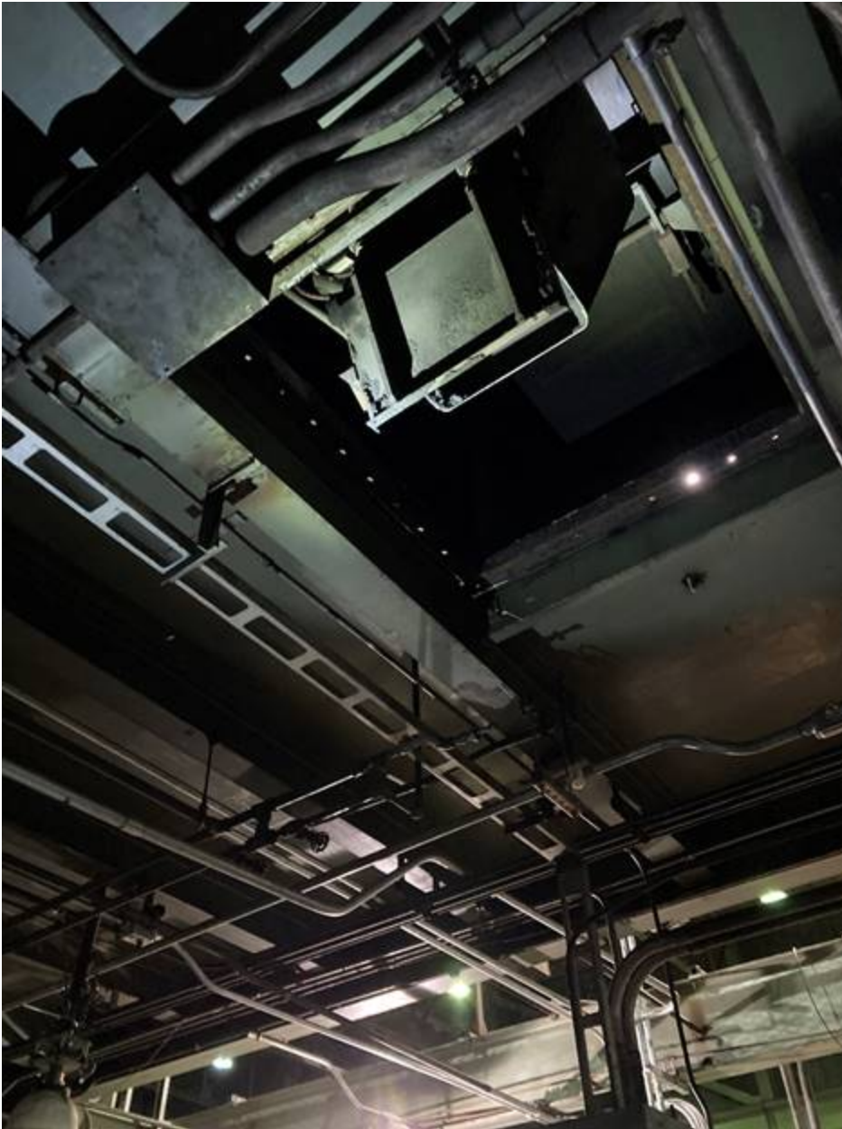
Image (1): Coal pulverizer equipment removed.
